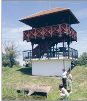
The lookout tower next to the bicycle path (VÁTI Nonprofit Ltd.)
