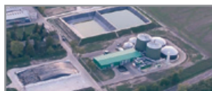
The view on the biogas plant ( www.greenfo.hu )
