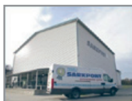
The refrigerating plant of Sarkpont Plc. ( www.sarkpont.hu )
