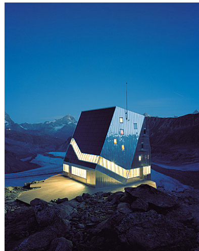
Figure 26: Autonomous rest house at the Monte Rosa, Switzerland
