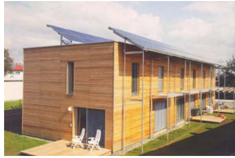
Figure 19: Passive house, Weiz, Austria
